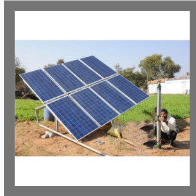
Solar Water Pump
